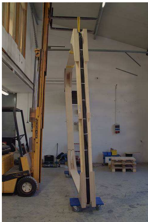
Lifting the coil with a forklifter
